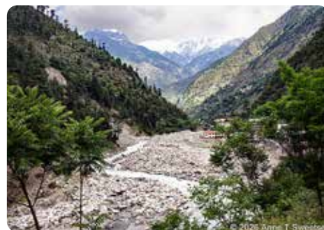
Flood damage half way up the Naran valley.
